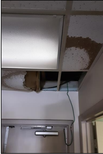
Example of Water Damaged Ceiling Tile
