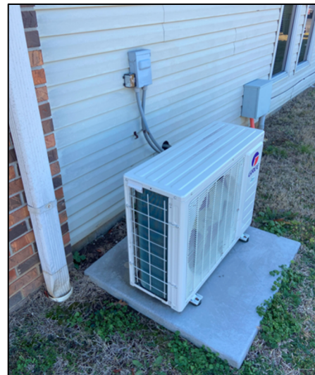
Figure M06. Radio Communications Outdoor Condensing Unit
