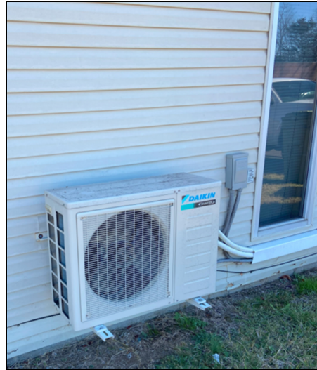
Figure M04. IT Room Outdoor Condensing Unit.
