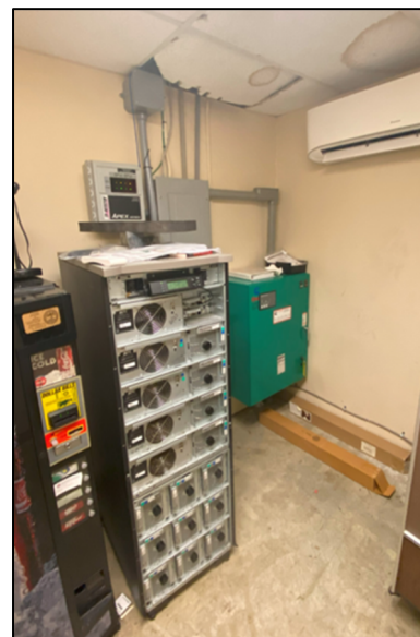
Figure E02. Existing Incoming Service, Automatic Transfer Switch, Main Distribution Panel, and IT Rack
