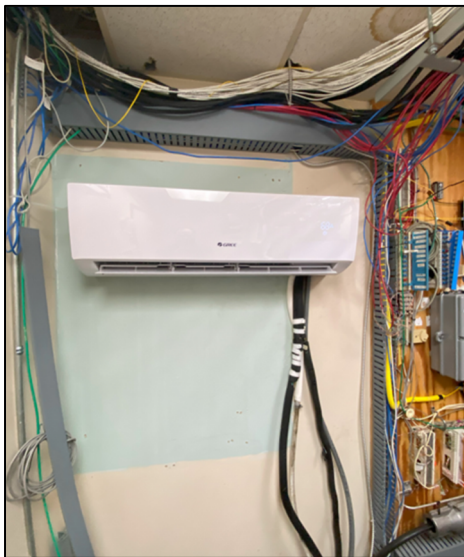
Figure M05. Radio Communications Indoor Wall Mounted Unit
