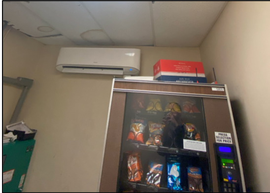
Figure M03. IT Room Indoor Wall Mounted Unit
